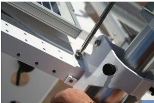
Use four 10-32 x 3/8" screws and a #2 Phillips to mount the DNI bracket to the side rail opposite the ShadowBand – two screws on top and two on the side.
