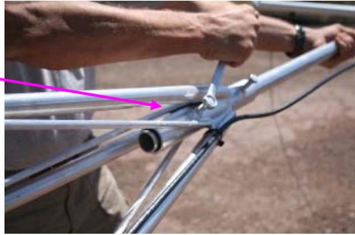
Begin threading the cable down inside the tower frame... run them along the rail opposite the grounding wire... there are some cable ties included, put one every five feet down to the top of the base section... there are several more cables to add to the bundle from there...
